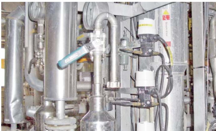
Robust field mount I/P converters for valve position control
