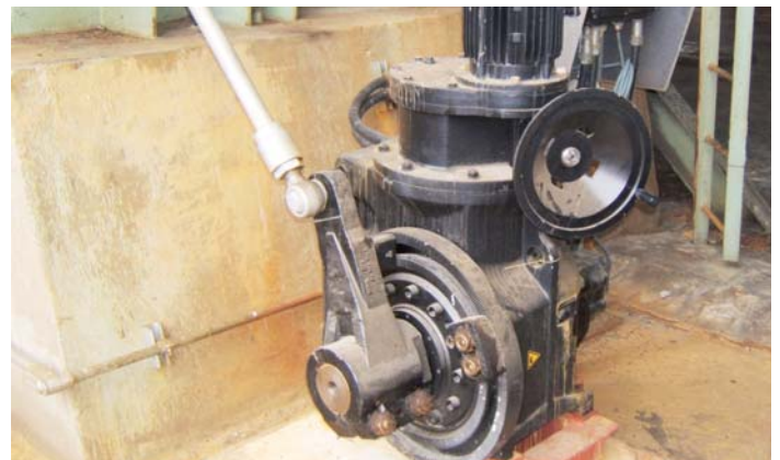
Actuator in forced draft fan control
